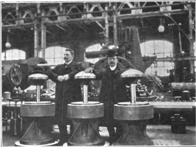
FIG. XIII. 65. Three Exhaust Valves for 2,000 H.P. Nürnberg Engine.
