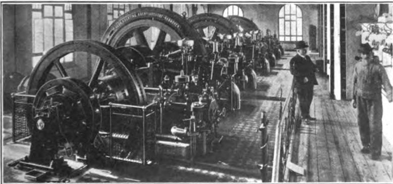
FIG. IV.—28. Six 300 H.P. Koerting four-cycle, single-acting, twin-engines at Julienhütte Electricity Generating Station.
