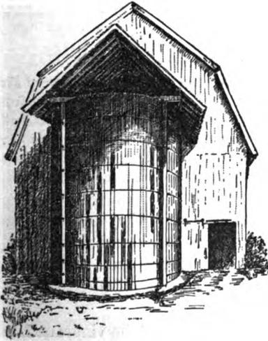
FIG. 178. A cheap roof of stave silo. (Clinton.)
