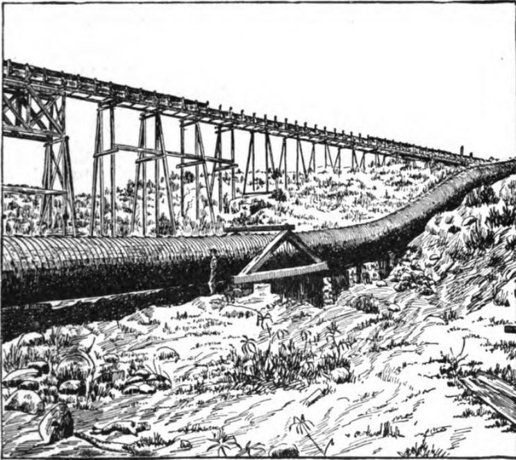
FIG. 28—STAVE PIPE-LINE IN POSITION.
