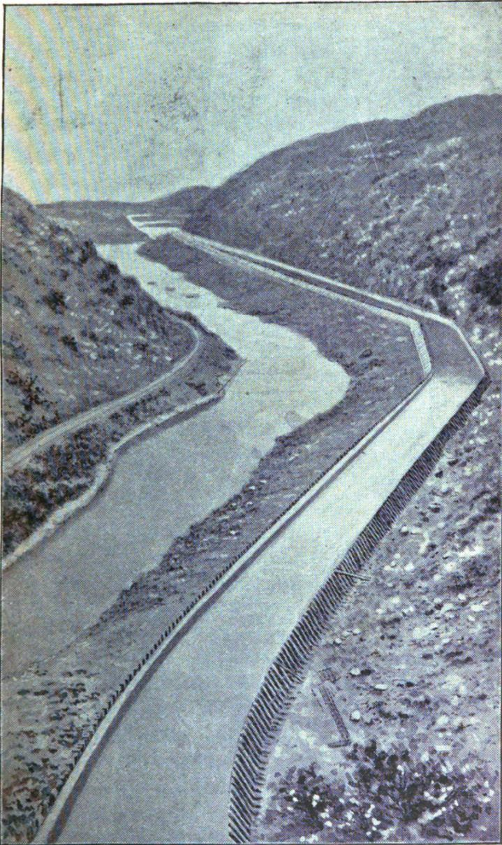
FIG. 33—BENCH FLUME FOR A LARGE CANAL.
